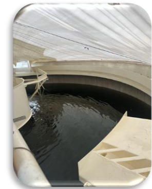
Secondary Clarifier No. 1 Recoating Project
