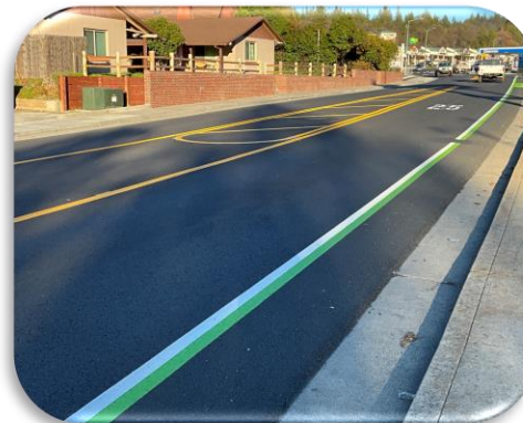
Broadway Sidewalks Project – New Sidewalk and Retaining Walls
